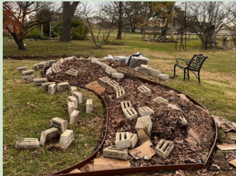
Vinyl edging in place and donated pavers ready to be installed
